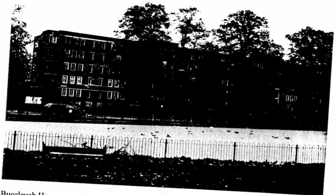
North elevation of Buccleuch House from Clapton Common
